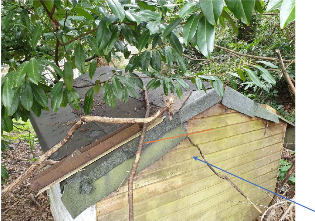
This picture has the laser level line transferred and projected from top of the fence along the boundary between 18 Parkside Road and 16 Parkside Road shown projected onto the back of the summer house.
